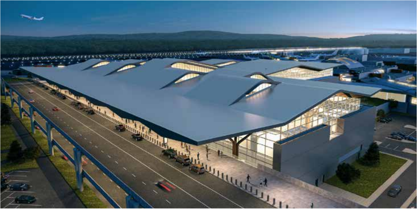
Local companies and expertise, led by architect Gensler and Luis Vidal, will be heavily involved in building Pittsburgh's new terminal.
