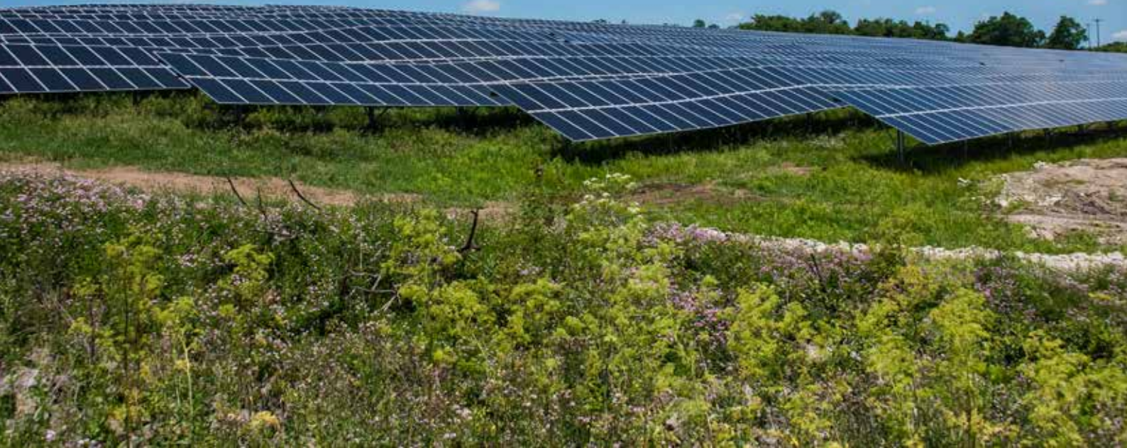
Pittsburgh airport now obtains all its power via a solar farm built on its grounds (all photos: Pittsburgh International Airport)
